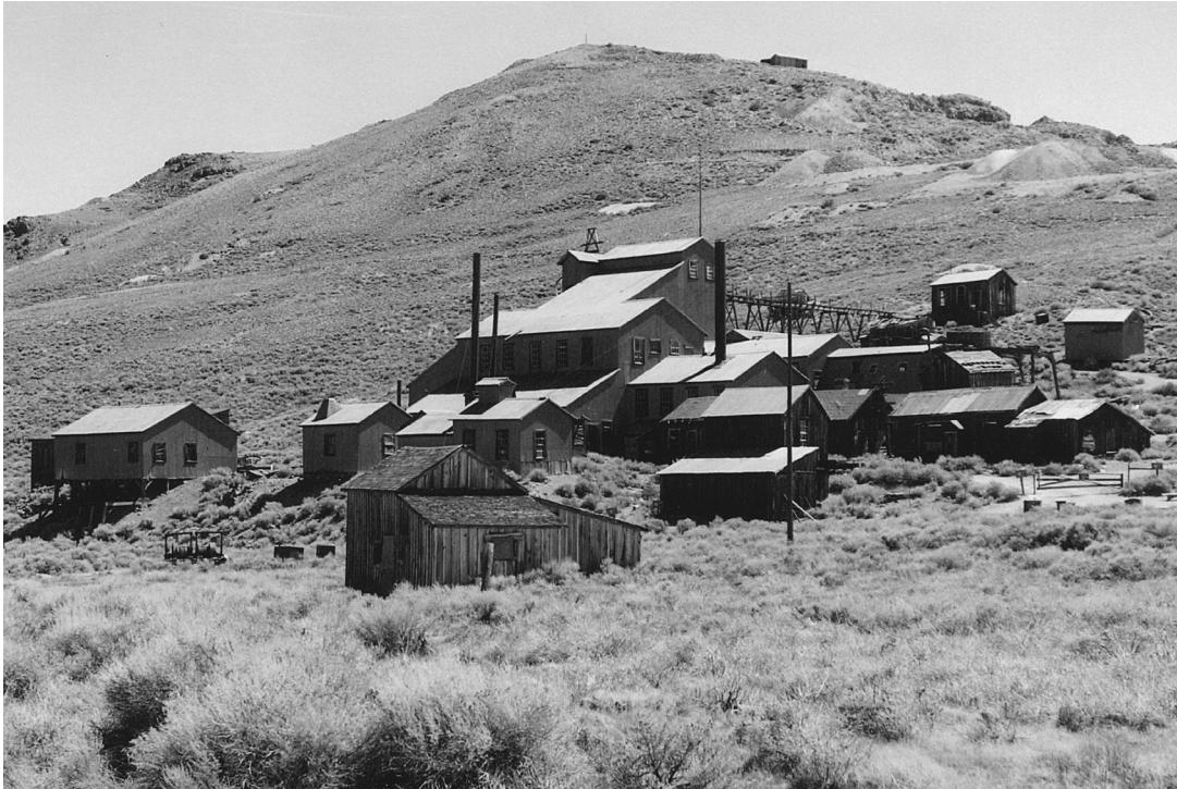
The second Standard Mill, a twenty-stamp California mill completed in 1899 to replace a similar plant destroyed by fire the previous year. These Standard mills were unusual in two respects: they were electrically powered and included a cyanide circuit housed in a separate building to the left (since destroyed) to reprocess the company's tailings.
