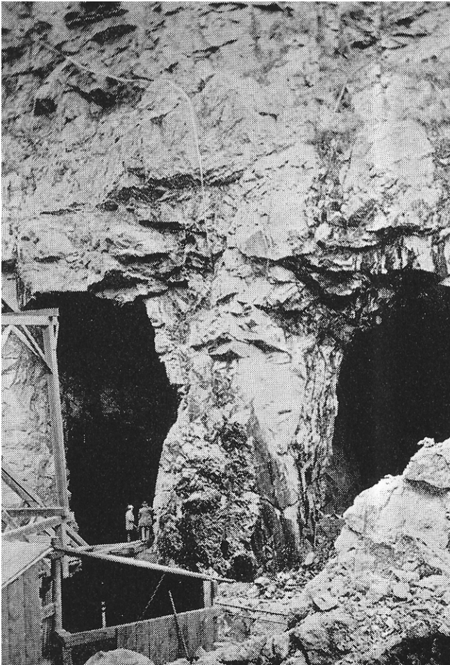
The Cleveland Iron Mining Company's Incline Mine, c. 1875. Note the size of the pillars left standing to support the overhang compared to the men standing at the left. The company had not yet adopted shaft mining and simply followed its ore deposit into the adjacent "mountain." (Cleveland-Cliffs Iron Company, The Cleveland-Cliffs Iron Company: An Historical Review of This Company's Development and Resources Issued in Commemoration of Its Seventieth Anniversary, 1850-1920 (Cleveland: Cleveland-Cliffs Iron Company, 1920), p. 11)
