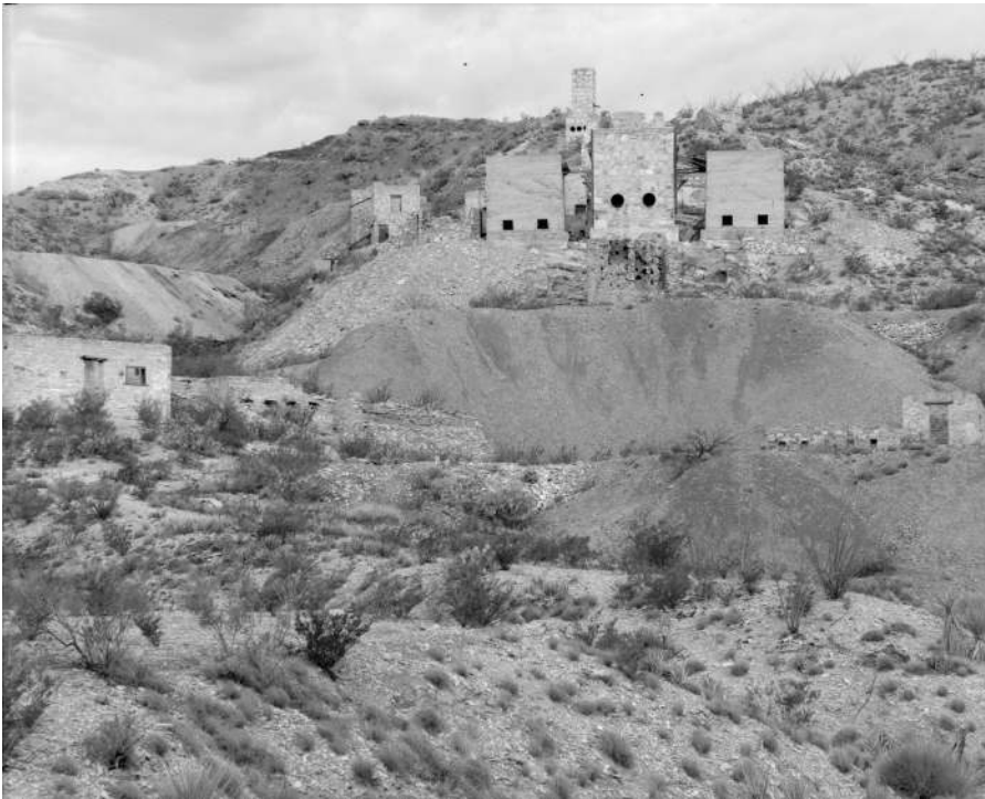
Three eras of mining activity on Mariscal Mountain are visible in this view. At the lower right are the Ellis era ruins; in the middle are the Mariscal era ruins; and at the upper left are the Vivianna era ruins. The mine entrance is at the top left. The piles of furnace tailings are prominent directly below the ruins of their associated eras. Photo by Bruce Harms.
