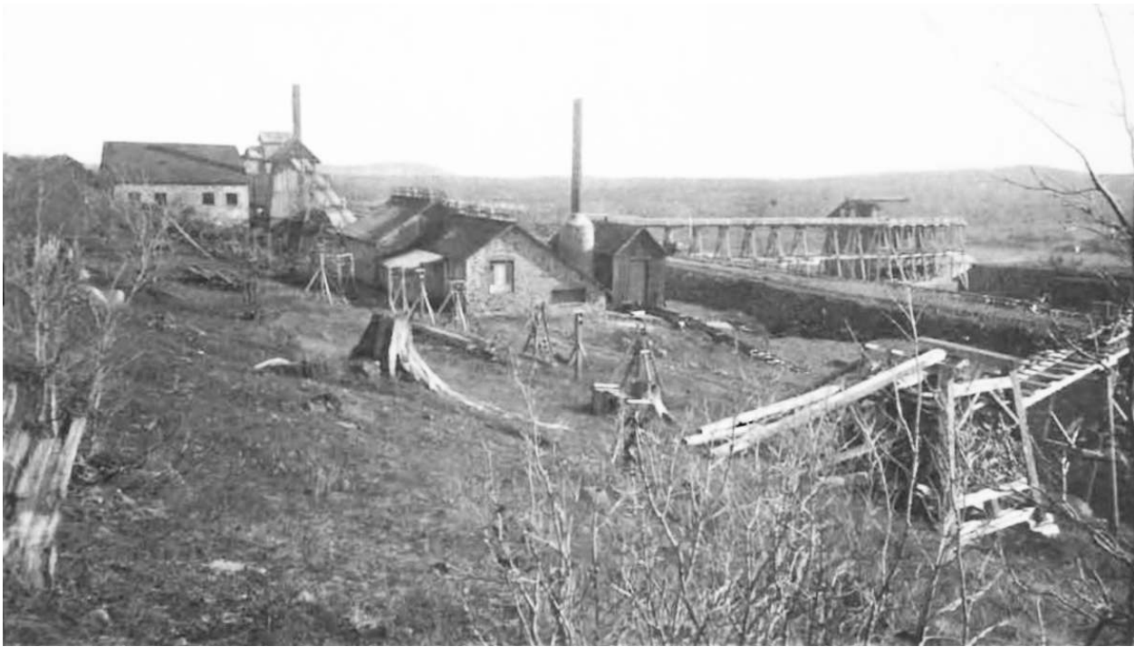
The North West Mining Company's engine house and shaft, constructed in the 1850s, are to the left of the smokestack in the center of this 1886 photograph. (From the prospectus "The Conglomerate Mining Company" (Philadelphia: The Company, 1887).)
