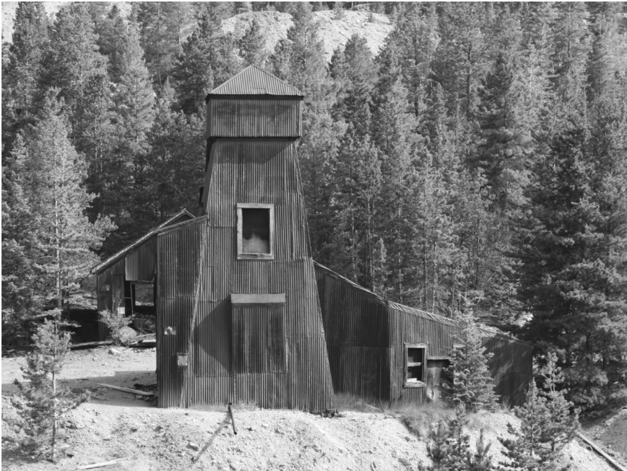
The headframe of the Pozo Mine at Nevadaville, Colorado. Placer mining began in Nevada Gulch, elevation 9,000 feet, during the earliest days of the gold rush of 1859, and it later became the site of some of the richest and deepest lode mines in "the Little Kingdom of Gilpin," as the county at the heart of early Colorado mining was known. (Editor's photo.)
