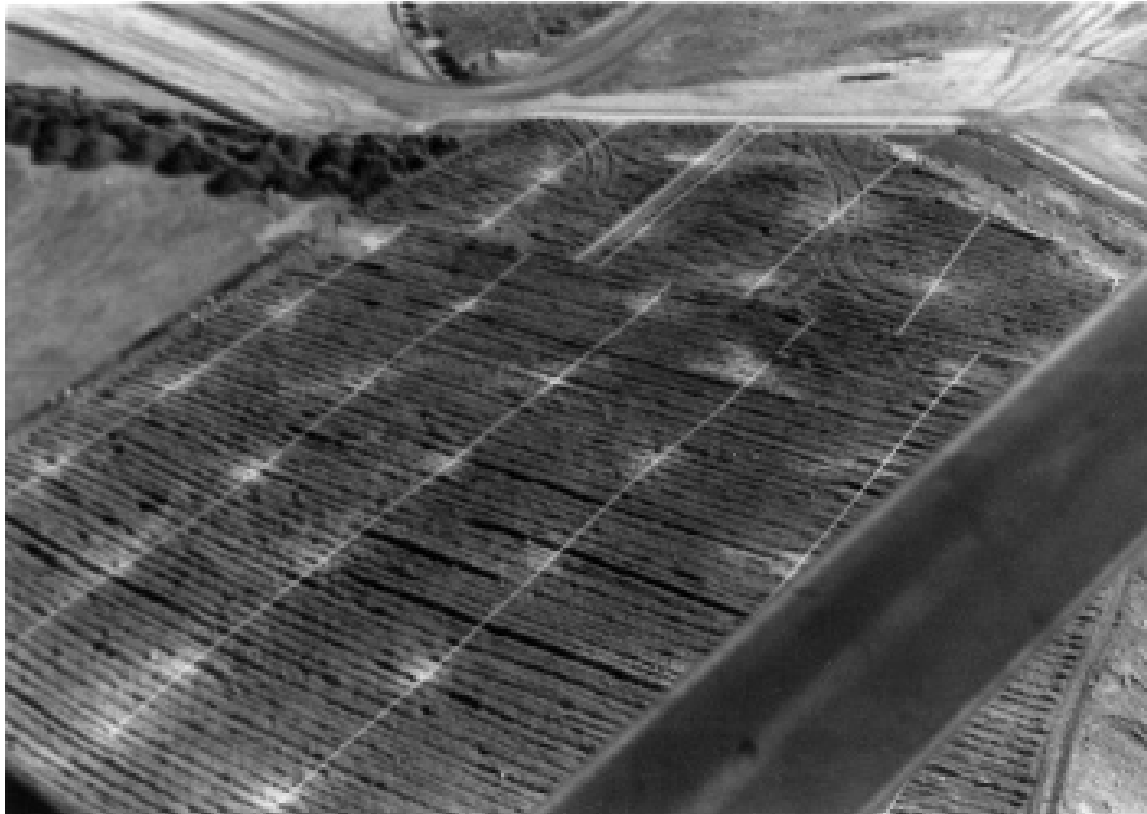
Aerial view showing the top of the heap-leach pad at Gold Acres, circa 1971, with its completed and very skillfully ripped surface, and sprayer lines in place. (Photo by Don Duncan courtesy of Lynn Duncan.)
