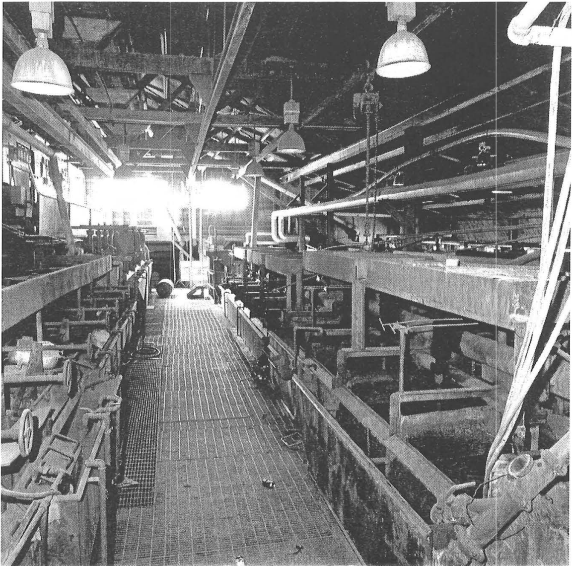
20-Cell No. 21 Minerals Separation Flotation. Interior of Shenandoah -Dives Mill, Silverton, San Juan County, Colorado, San Juan County Historical Society, Silverton, Colorado
