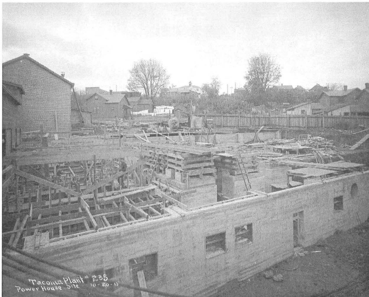
Figure 6 Power House, Tacoma Plant, with houses nearby.
