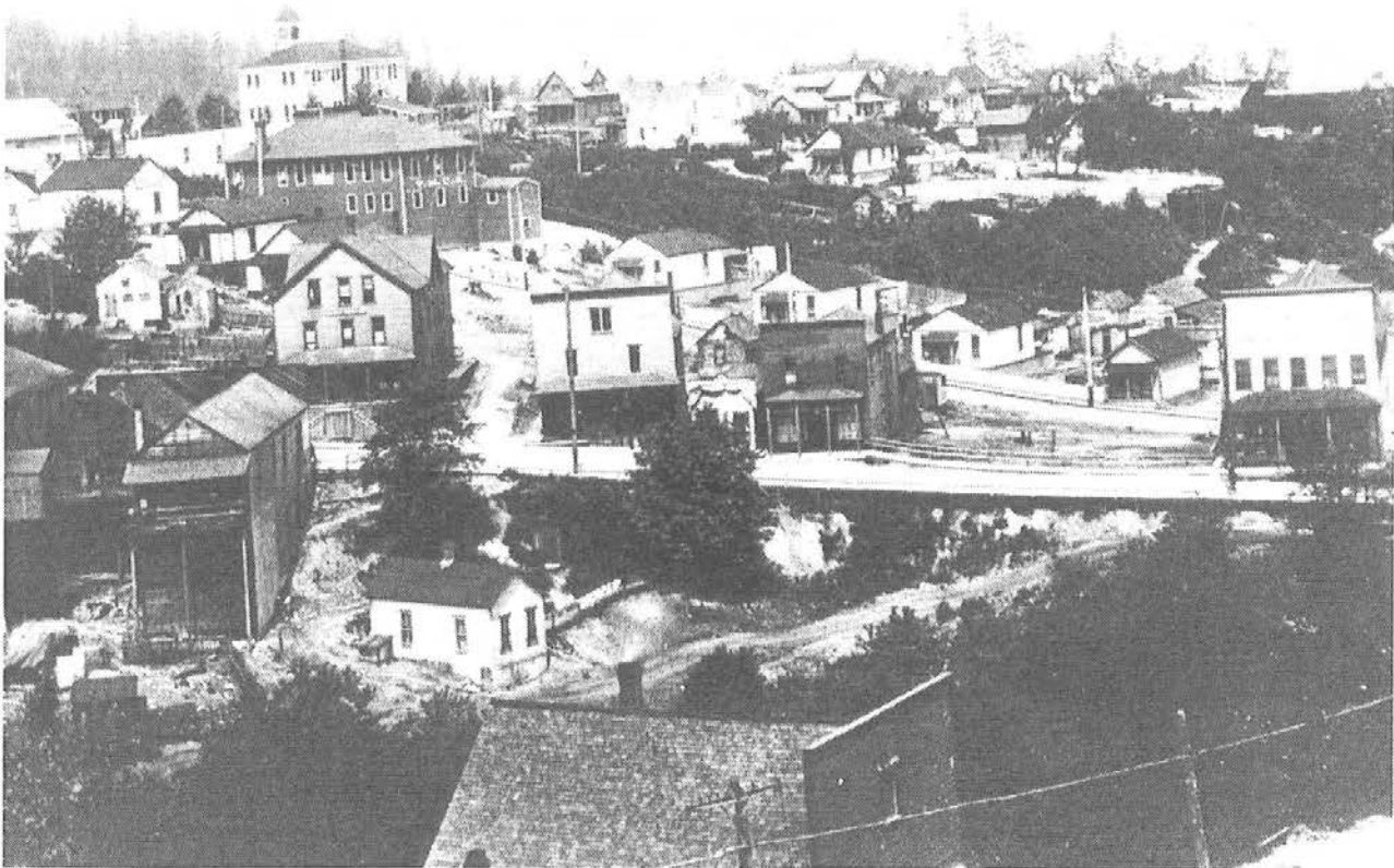
Figure 5 Hillside just outside smelter gates about 1890.
