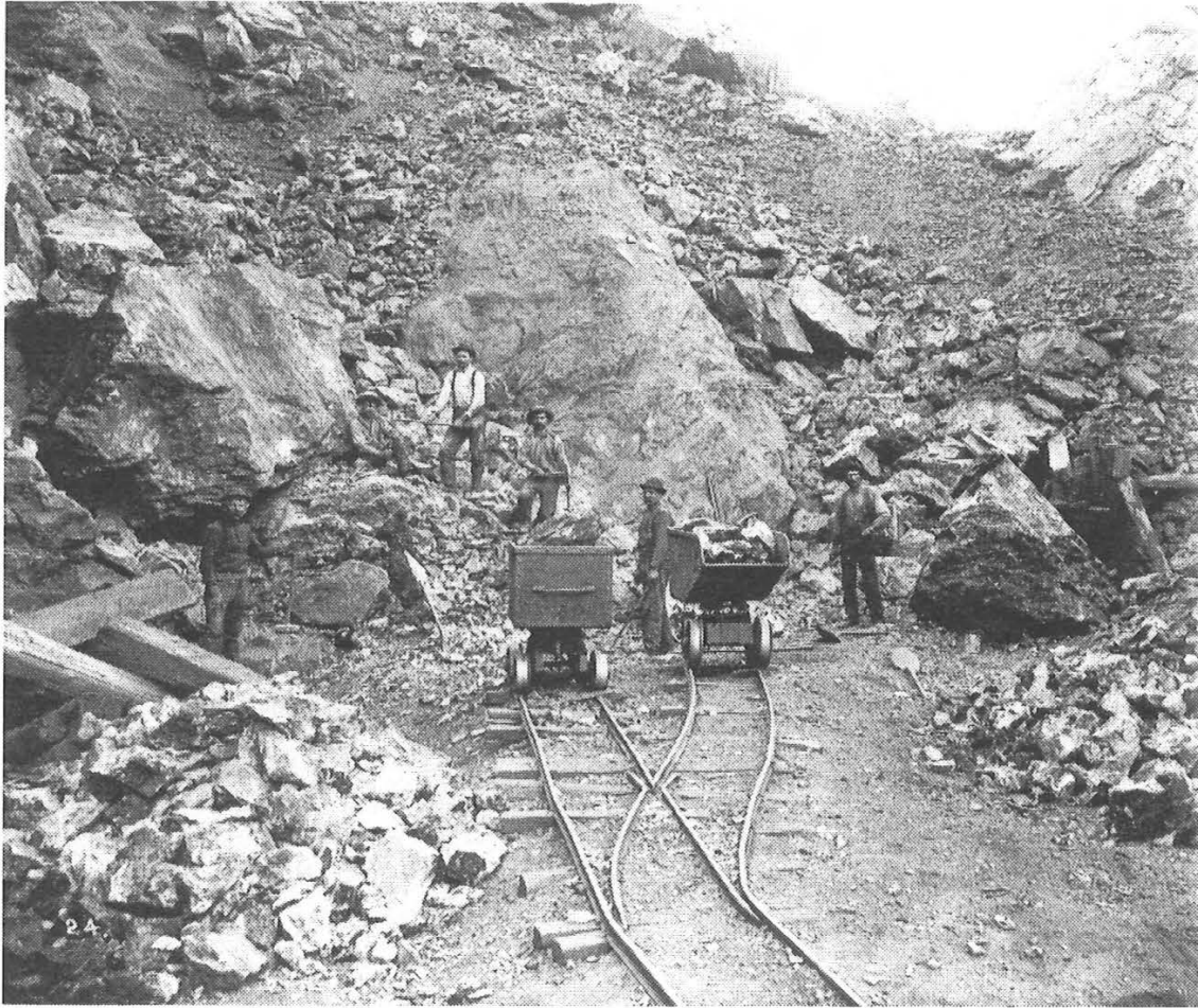
Figure 1 Hand drilling blastholes at the Bunker Hill discovery outcrop. Circa 1886. #8-x24, Historical Photograph Collection, University of Idaho Library, Moscow, ID
