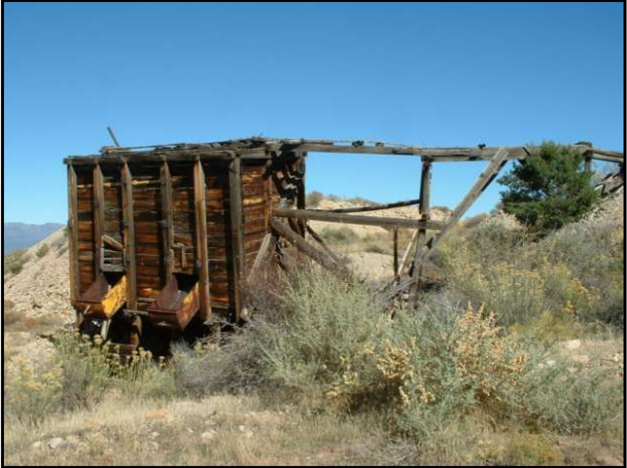
Figure E 5.15. Capitalized mining companies often erected formally designed and well-built sloped-floor bins, such as the one at the Republican Mine in Long Park. Miners input ore by pushing ore cars across the trestle and dumping them directly into the bin. A truck parked underneath the chutes to receive loads of ore for shipment. The sloped floor allowed the ore to pour into the truck with minimal handling. Source: Author.
