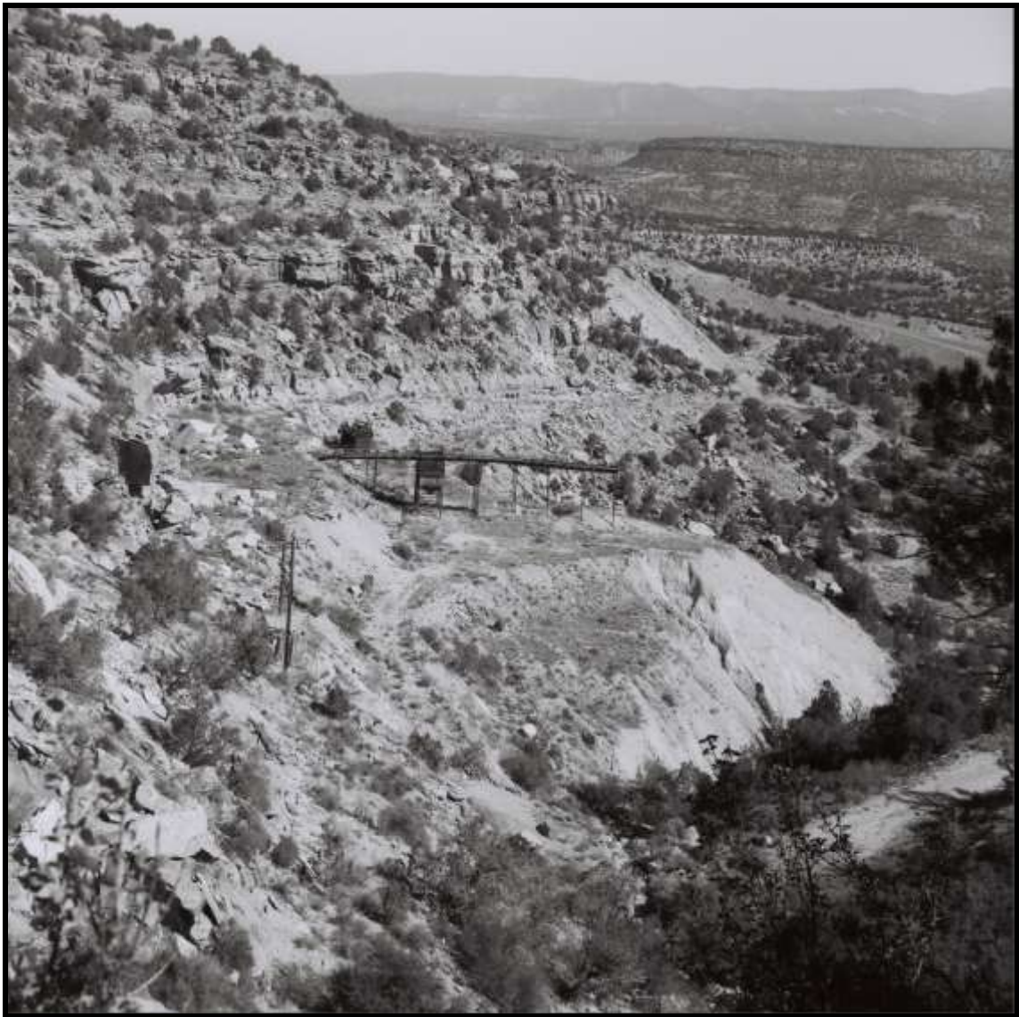
Figure E 5.6: The Rex No.38 Mine in Eagle Canyon is a sound example of a tunnel operation. Distinguishing characteristics include a lengthy tunnel, a voluminous waste rock dump, an ore bin, and a trestle. Source: Author.
