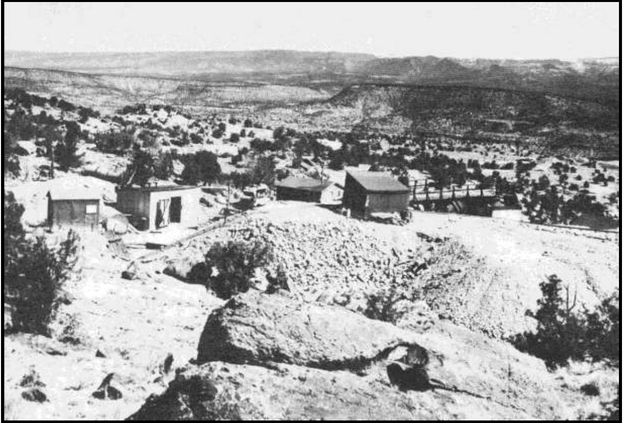
Figure E 5.9: The photo illustrates a surface plant typical of medium-sized and large mines. The mine in the photo may be either a horizontal or inclined tunnel operation. The surface plant features several frame buildings, an ore bin and trestle, and a portable air compressor. Note the small sizes and simplicity of the buildings, which appear to be of frame construction sided with tarpaper. Dare, 1955:22.
