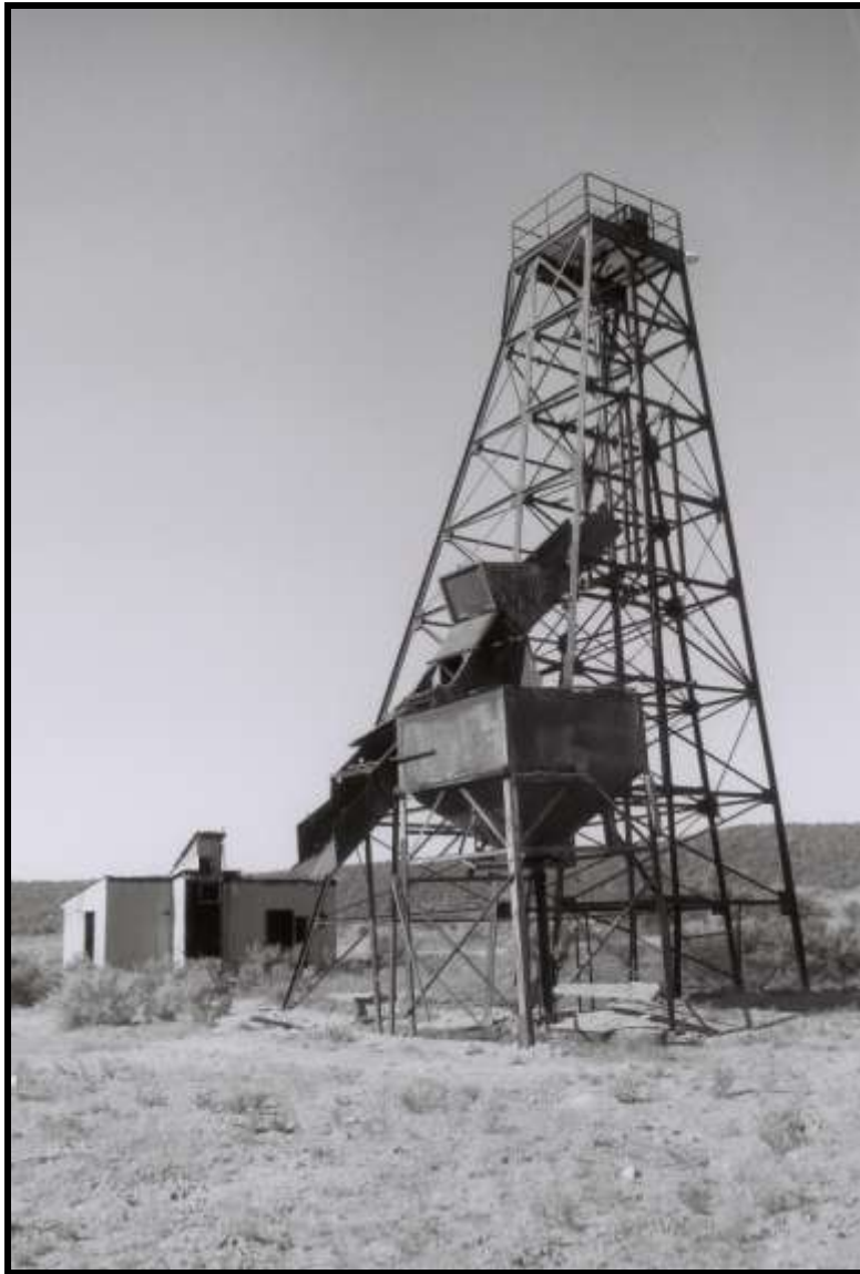
Figure E 5.8: The Long Park No.1 Mine is an excellent example of a large, formally engineered vertical shaft dating to the 1950s Cold War uranium boom. The mine features a lofty four-post derrick steel headframe, a frame hoist house, and a factory-made ore bin. A skip hoisting vehicle automatically dumped rock into the chute. If the material was ore, a swinging gate diverted it into the bin. If the material was waste rock, it accumulated on the ground and then was bulldozed away. Source: Author.
