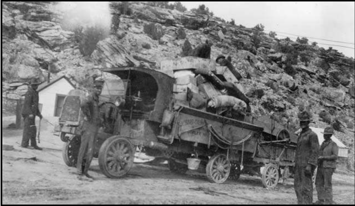
Figure E 5.1: This 1910s diamond drilling crew embarked for a lengthy exploration campaign in Montrose County. The truck and trailer carried camp supplies and drilling equipment. The amount of capital required for drilling limited this exploration method to the region's large companies. Source: Denver Public Library, Z-7844.
