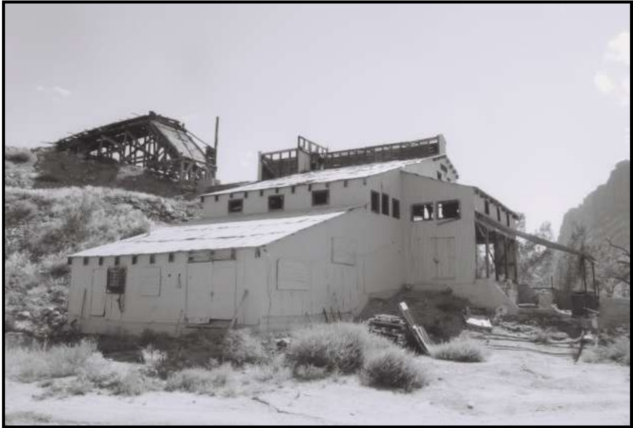
Figure E 4.7: The Gateway Alloys mill began recovering vanadium from carnotite ore in 1939. By accepting ore from independent companies, the mill directly supported mining in Montrose and Mesa counties. Source: Author.
