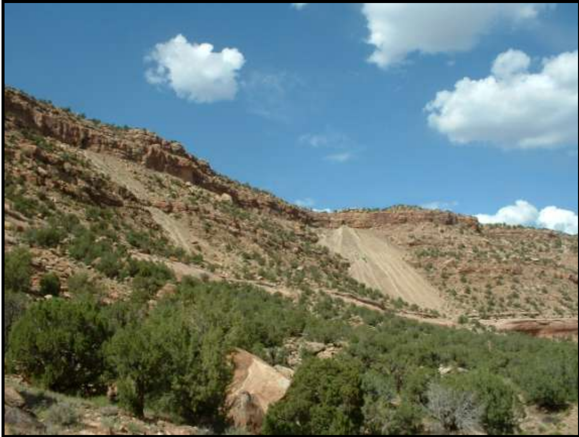
Figure E 5.5: Rim mines were so named because they were developed in the sandstone cliffs, or rims, of the region's mesas. As the photo illustrates, rim mines were confined to the same horizontal beds, were relatively limited in size, and were developed through tunnels. Source: Author.
