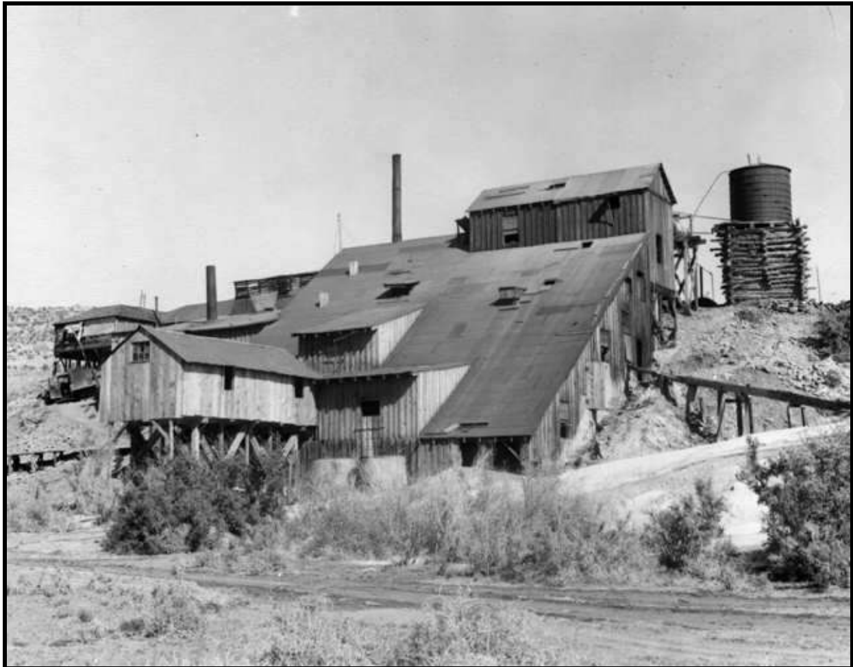
Figure E 4.2: The Rare Metals Mill, built in 1903, was North America's first commercial uranium concentration facility. A succession of companies operated the mill, which apparently burned during the 1920s. The exact date of the photograph is unknown, although most likely during the 1910s. Source: Denver Public Library, X-61965.
