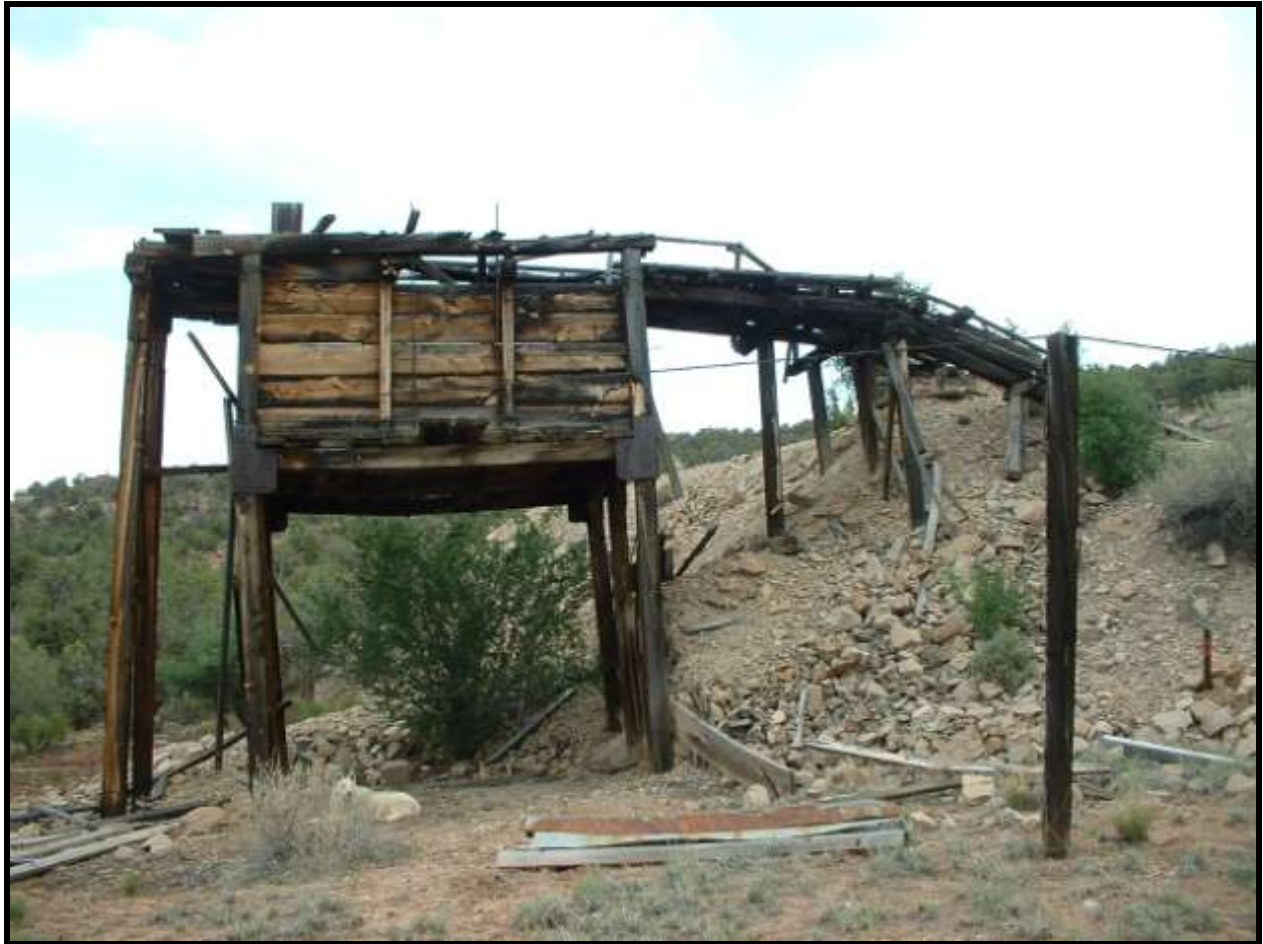
Figure E 5.16: Most uranium mines featured simple flat-bottom ore bins, such as this example at the Margie Mine on Club Mesa. The bin is a little more than an elevated box constructed with salvaged materials and no formal support system. A truck parked underneath to receive ore for shipment. Source: Author.
