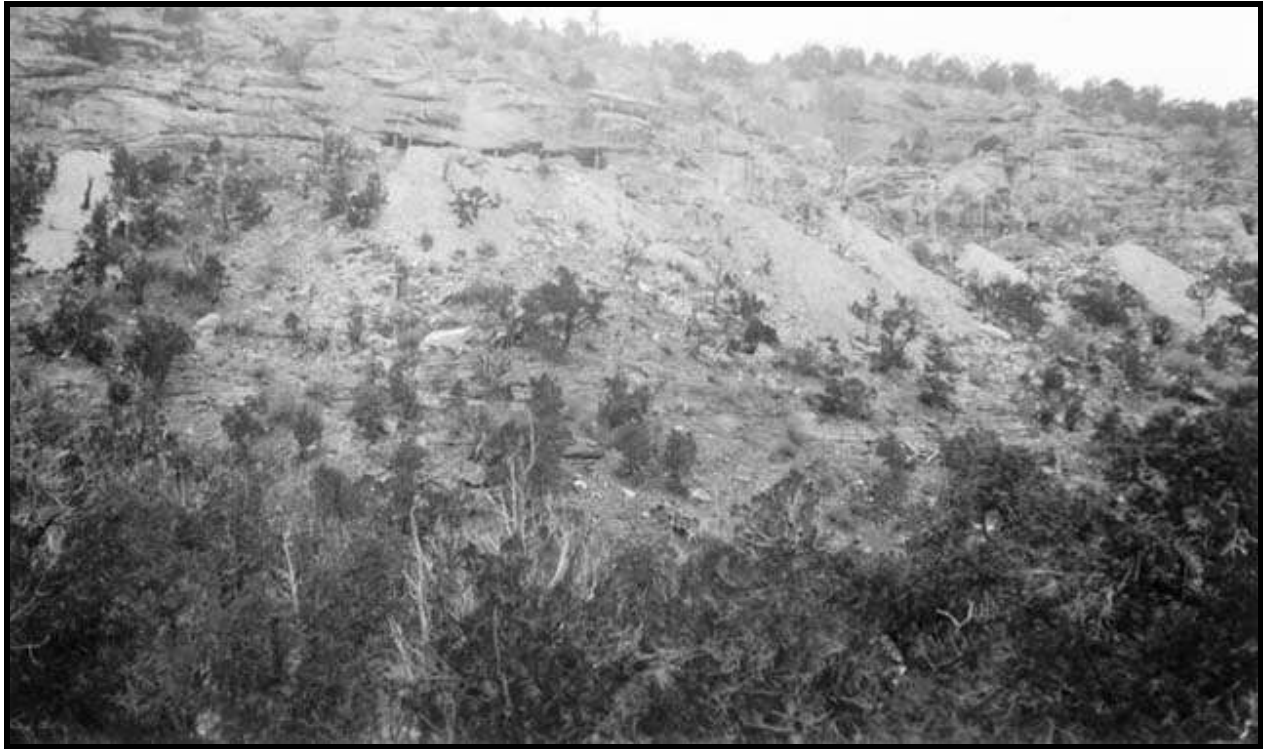
Figure E 4.1: Because carnotite beds cropped out in the cliffs of the region's mesas and river valleys, they were easy to access and hence required little capital to work. The photo illustrates one of the many small mines developed during the 1900s. Source: Denver Public Library, CHS.X5629.
