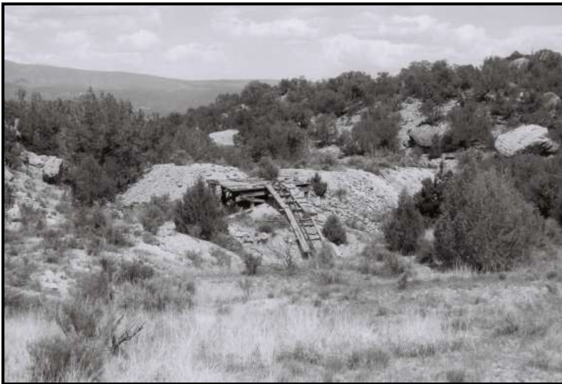
Figure E 5.7: The Donna K Mine exemplifies a typical inclined shaft site. An inclined trestle ascends out of the shaft and terminates on a hoist frame. The trestle carried a track that forked on the substantial waste rock dump, and one branch extended to an ore bin while the other ended on the dump. Miners parked a portable air compressor, now gone, to the right of the shaft, and a frame hoist house stood on the hoist frame. Source: Author.
