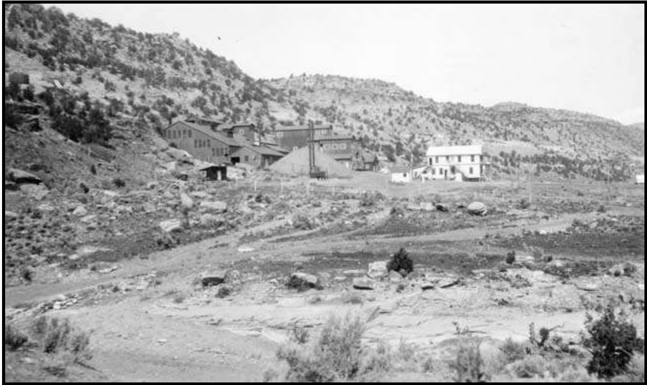
Figure E 4.5: View west of the Standard Chemical Company mill and boardinghouse during the late 1910s. The mill was critical to uranium and vanadium mining in Montrose County because it offered local ore treatment. The mill was among the nation's largest uranium concentration facilities. Source: Denver Public Library, CHS.X5634.
