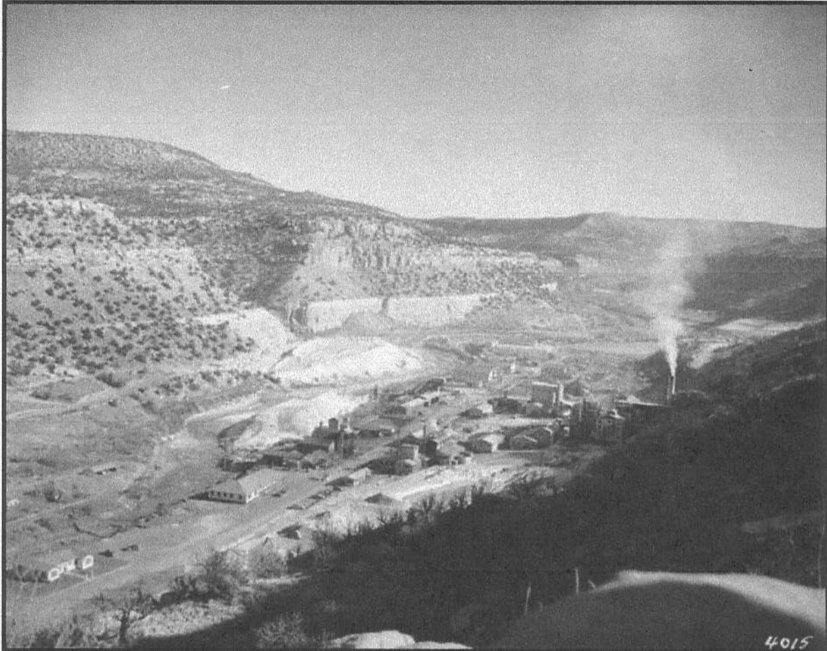
Figure E 4.9: This easterly overview shows how large and complex United States Vanadium's Uravan Mill was during World War II. The mill recovered vanadium from crude ore for armor and weapons, and, under secrecy, uranium for the Manhattan Project. Source: Denver Public Library, CHS.X6203.
