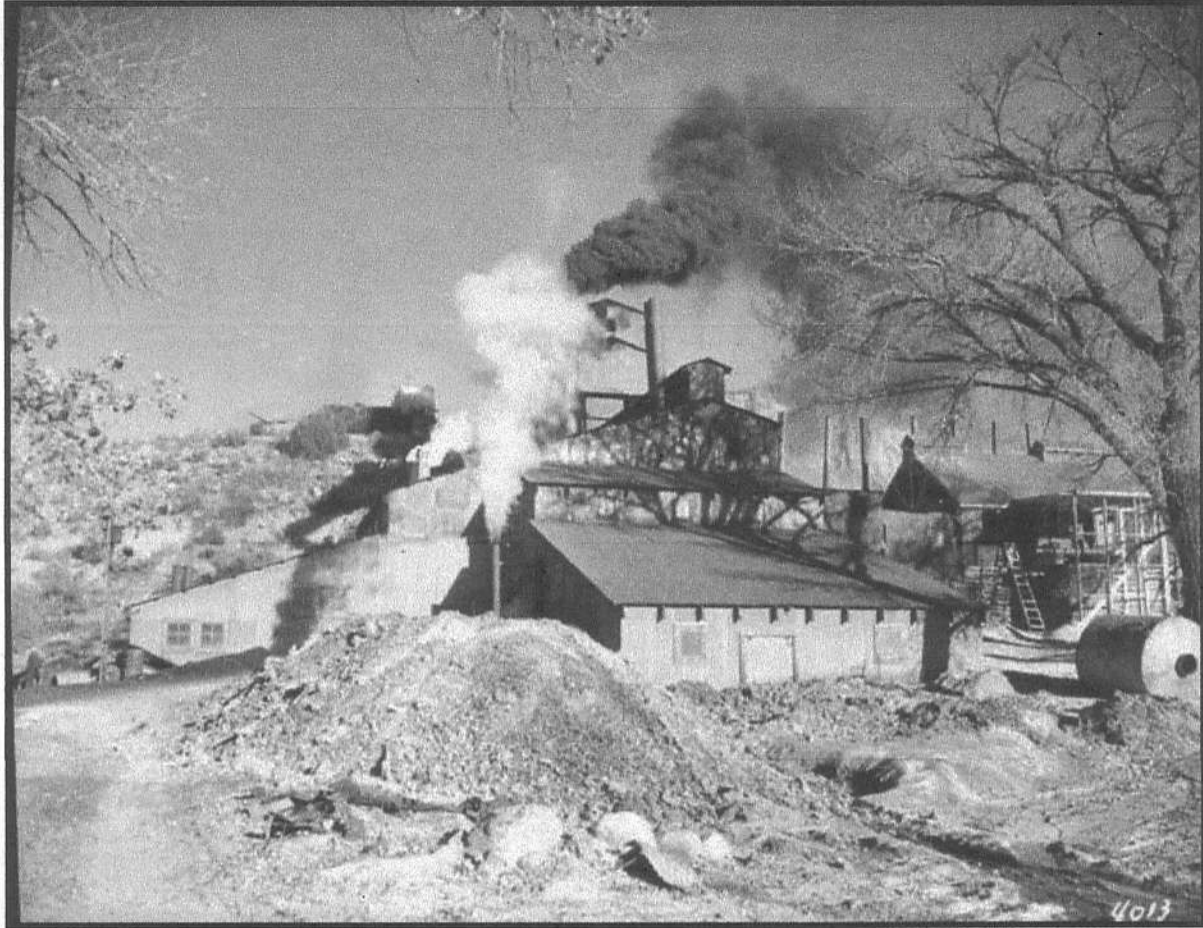
Figure E 4.10: During World War II, the Vanadium Corporation of America operated its mill at Vancorum. The mill was built in 1930 to recover vanadium from crude ore, and it stood idle until the Vanadium Corporation of America started it during the late 1930s. During the war, the facility not only produced vanadium as designed, but also recovered uranium from crude ore and tailings brought in from other mills. Like the Uravan mill, the uranium operations were secret. Source: Denver Public Library, CHS.X6201.
