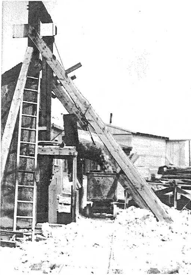
Fig. 16 Wade Shaft No. 2. Note bucket dump. This undoubtedly fractured otherwise usable crystals.
