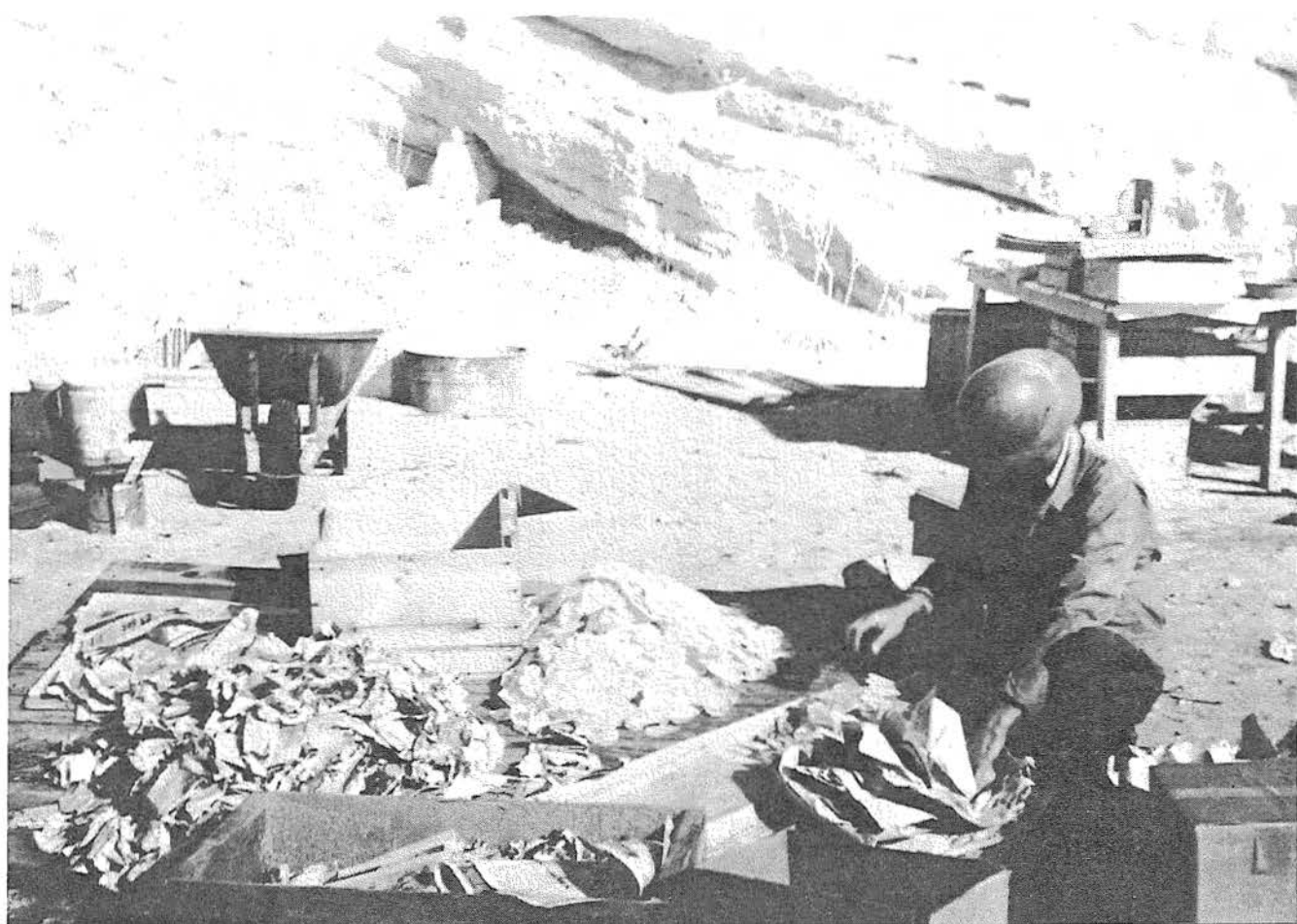
Fig. 8 Jack Frost packing crystals for shipment at Palm Wash. Inspection table and acid wash equipment in background. Courtesy Phil Blazovic.
