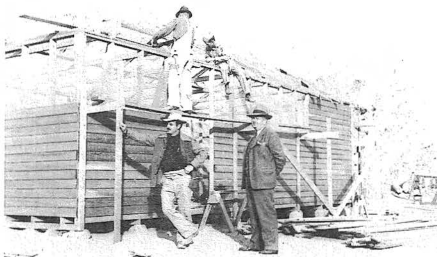
Fig. 10 Arnold Hoffman and Paul McCulloch supervise construction of building at Palm Wash mining camp. Note Marine helping carpenter. Courtesy McCulloch.
