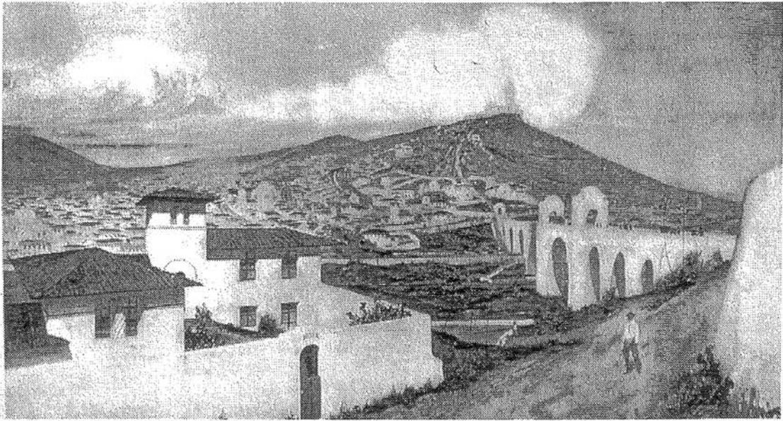
Fig. 6. Elliott designed the large aqueduct, seen on the right, to replace an existing flume that transported water from the mines to serve agricultural lands. The aqueduct also carried a roadway that connected two hills, and functioned as a "city gate." "The Aqueduct and Town, from the Western Hill of the Gap," from a drawing by Huger Elliott in "An Ideal City in the West," *The Architectural Review* (September 1908), 138.
