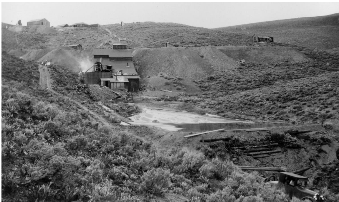
This 1932 photo shows the mill building, tailings pond and other mine buildings of the Big Six. The tall building in the upper left corner of the photo is likely the headframe for the Big Six inclined shaft. (Photo from Northern Nevada Field Trip notes of A. M. Smith and C. Stoddard 1932, used by permission of Special Collections, University of Nevada, Reno)
