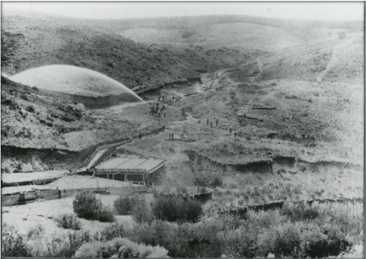
Hydraulic mining at Gold Creek, Nevada, 1897. Photo courtesy of Northeastern Nevada Museum, Elko
