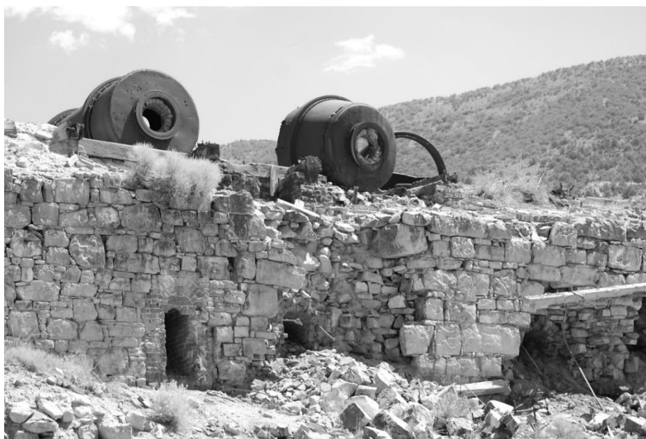
Tenabo Mill ruins including two Bruckner furnaces on top. The flues under the furnaces are lined with brick made locally in Grass Valley. Photo courtesy of Robert McQueen.
