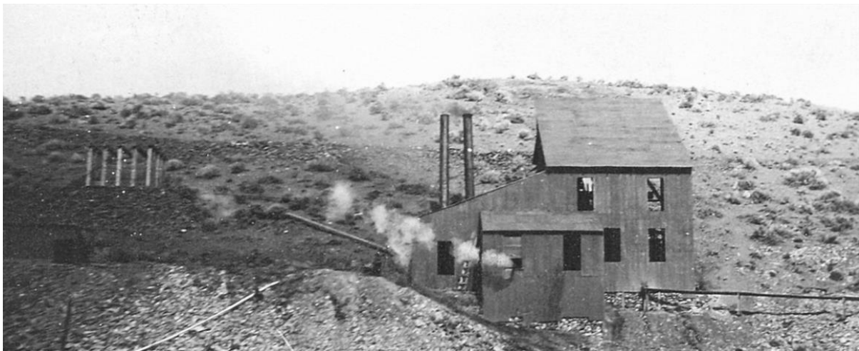
One of the first mills in the Gold Circle Mining District, this 10-stamp facility was built by Charles L. Geyman (of Butte, Montana, fame) in 1908. It was usually operated by his wife, Josephine Chishart Geyman until about 1921. She had become nationally famous for operating the Yankee Boy Mine and Mill in Butte while Charles was imprisoned in 1905. Photo courtesy of Friends of Midas.
