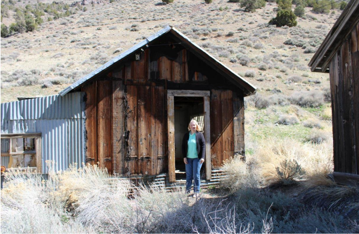
Kaye Shelley in front of schoolhouse, April 6, 2022.
