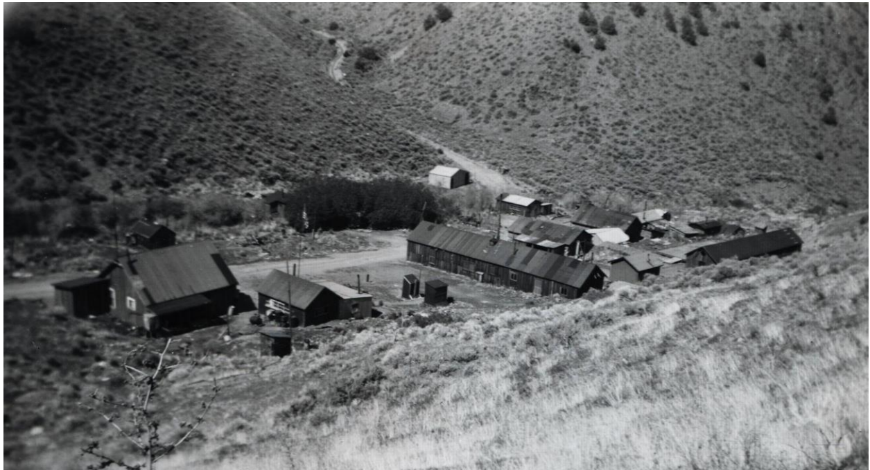
View of Mill Canyon settlement. Superintendent's house (far left) with school and attached teacher's house. Possible barracks on right. (not identified in Nile's photos)
