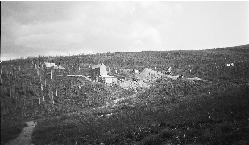
Rhoads-Hall Mill under construction, 1911 (it would later become Cleary). Cornell University Library
