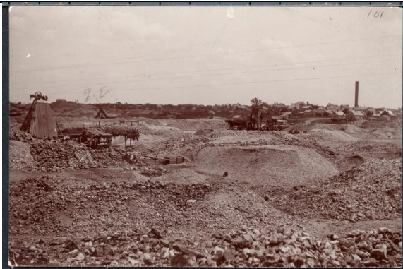
Hazardous subsidence resulted from the extensive shallow mine workings and 377 abandoned shafts in Galena, KS. The area in the photo was dubbed "Hell's Half Acre."
